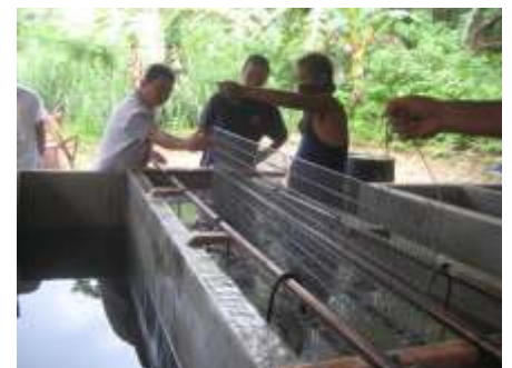
MIRDC consultant for Electroplating conducts trial run of the Electro Galvanizing facility set up for Egger Farm.
