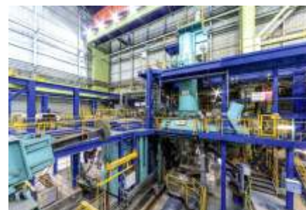
Production of specialty steels and super alloys at Tata Steel in Stocksbridge, using the new VIM X-eed® unit supplied by SMS group
