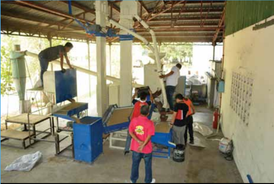
Setting-up of retrofitting machineries at PHILMEC, Nueva Ecija.
