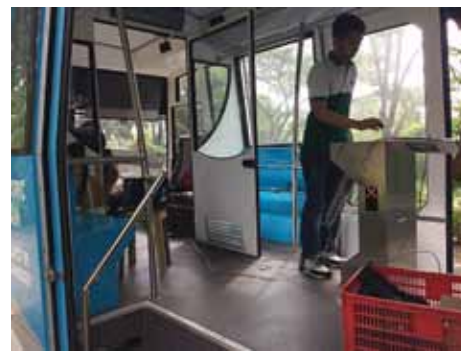
Ticketing System Installation of CRT.
