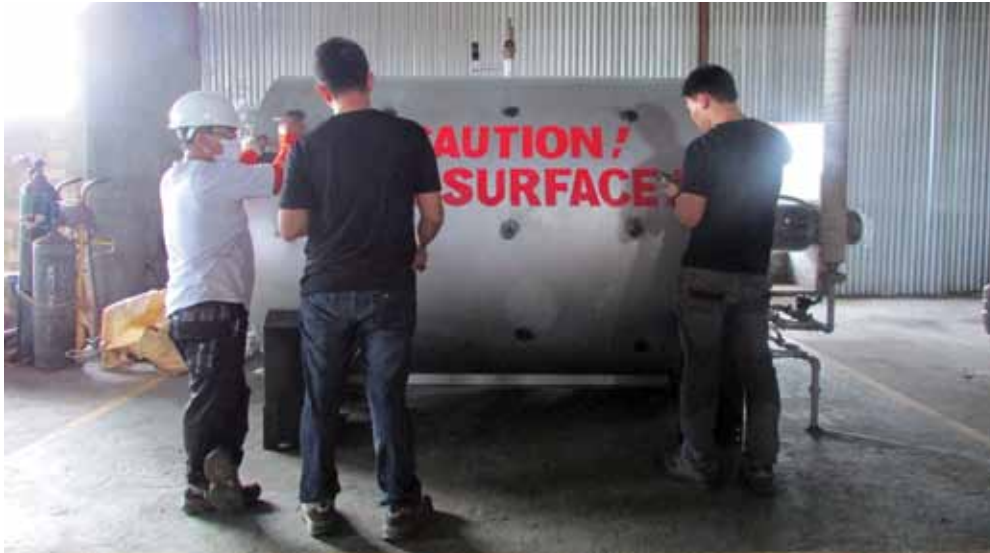
NDT personnel ANPilar, JABCabarloc and AYVPacia check the weld area and measure the thickness of a boiler in a chemical plant.
