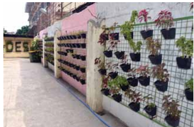
The steel matting frames used in the vertical garden of the Daang Hari Elementary School, fabricated and installed by the MIRDC.
