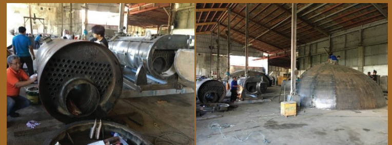
NDT staff conducting PT on Boiler Housing
