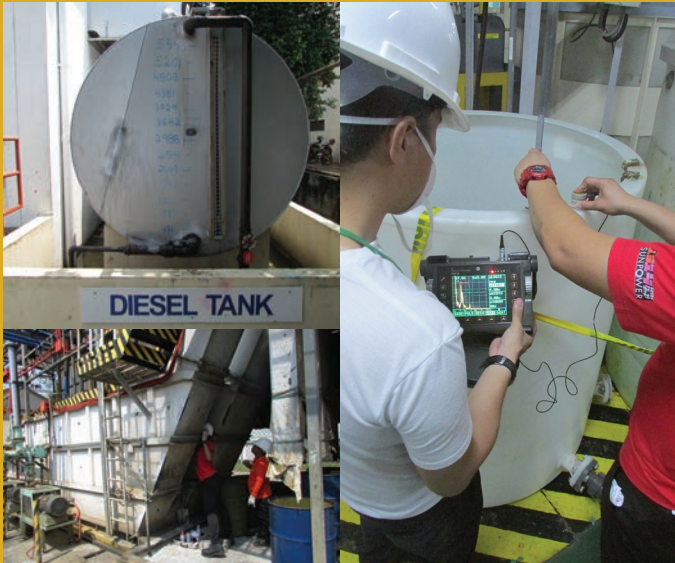
Integrity test on Tanks
