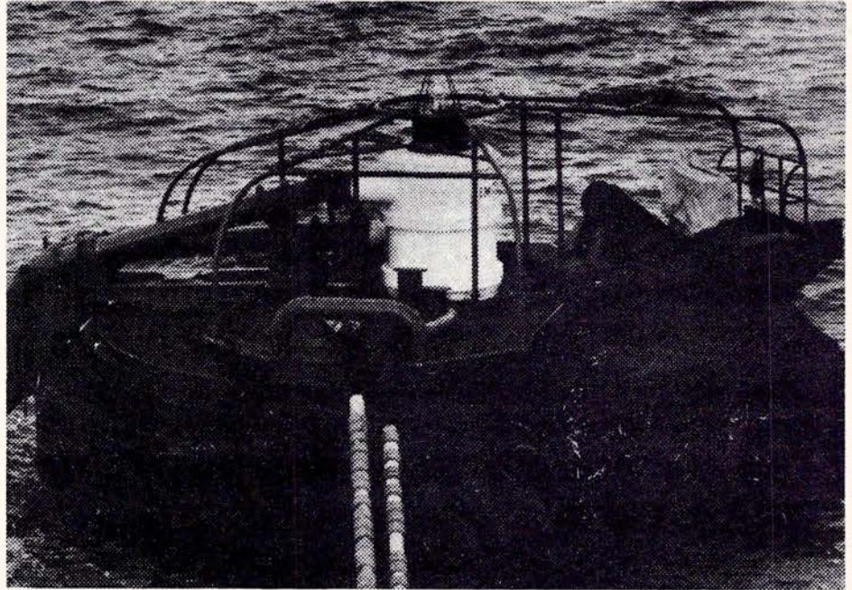
Anchored one and one-half miles off New Zealand's North Island, buoy above serves as critical transfer point in submarine pipeline from iron sands mines ashore and as mooring facility for large ore carriers operated by Marcona Corporation, USA.
