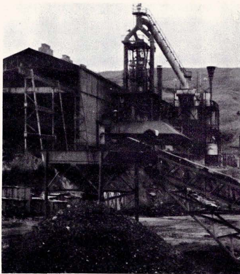
A general view of the NASSCO-J. Panganiban low-shaft furnace and casting hall from the ore stock yard.
