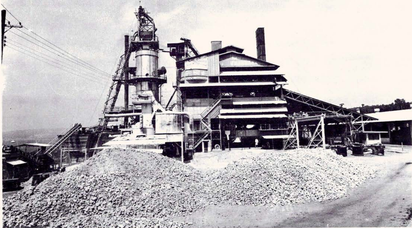
Profile of carbide plant in Iligan City. The cylindrical structure at left is the lime kiln. The main building at right house the furnace (with stack) and packing division. Foreground show limestone stockpile.
