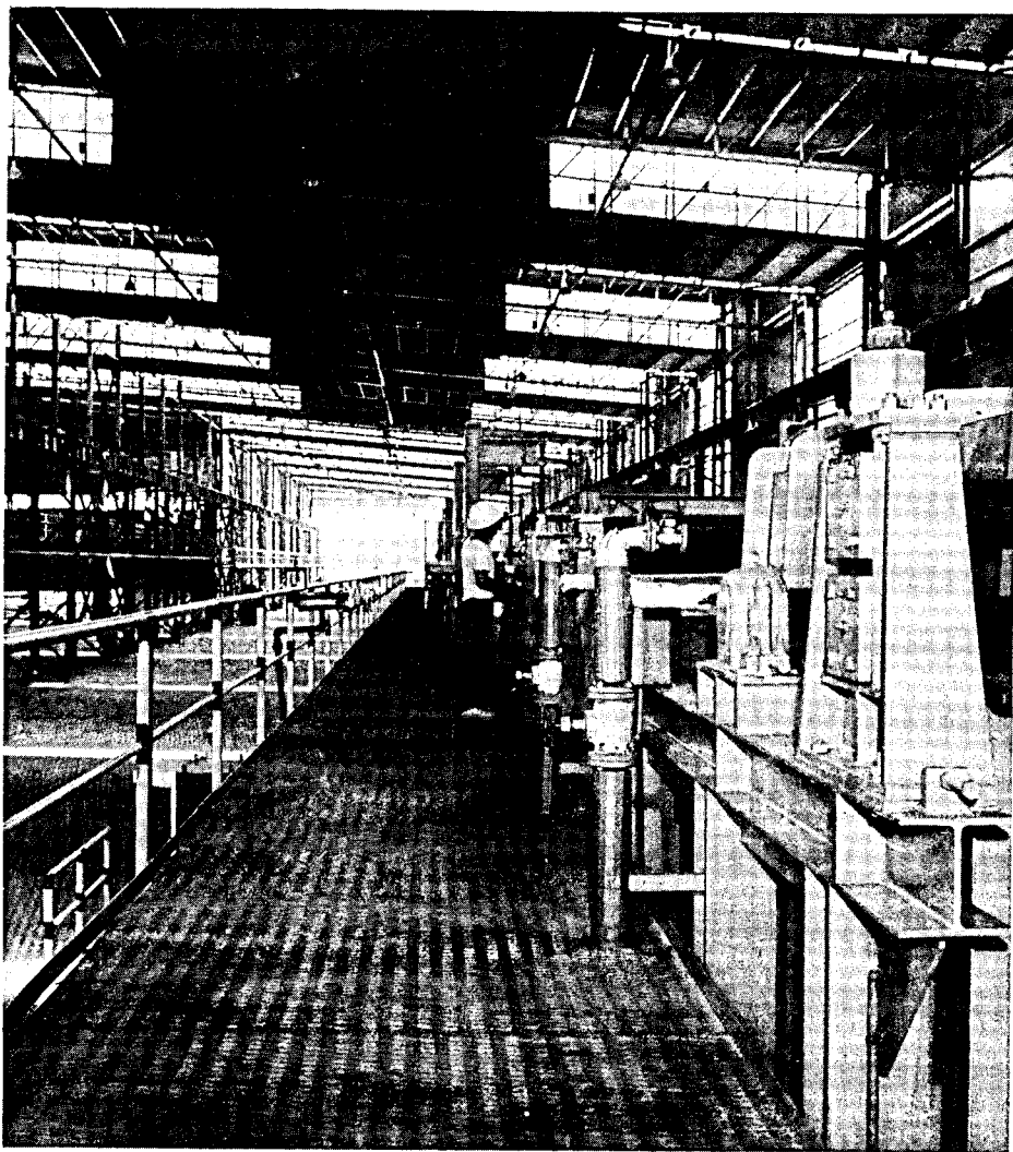
Photo shows the delivery section of the continuous pickling line. Hot bands undergo first major processing in this section.
