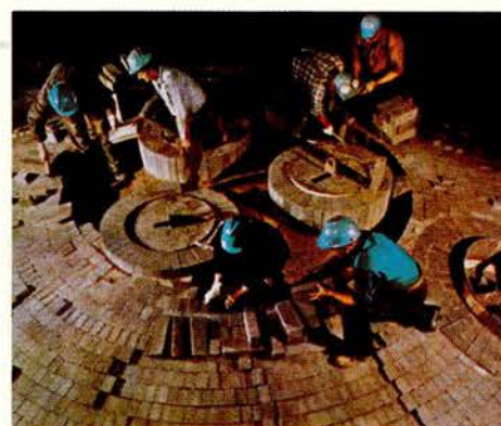
Installing an arc furnace roof lining of Alro 80 refractories.
