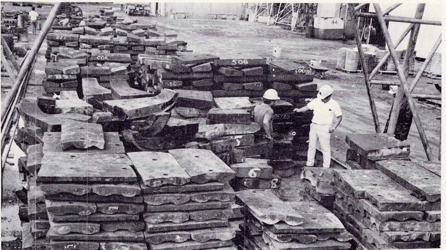
Ball mill liners are stacked in storage yard adjacent to the steel foundry building.
