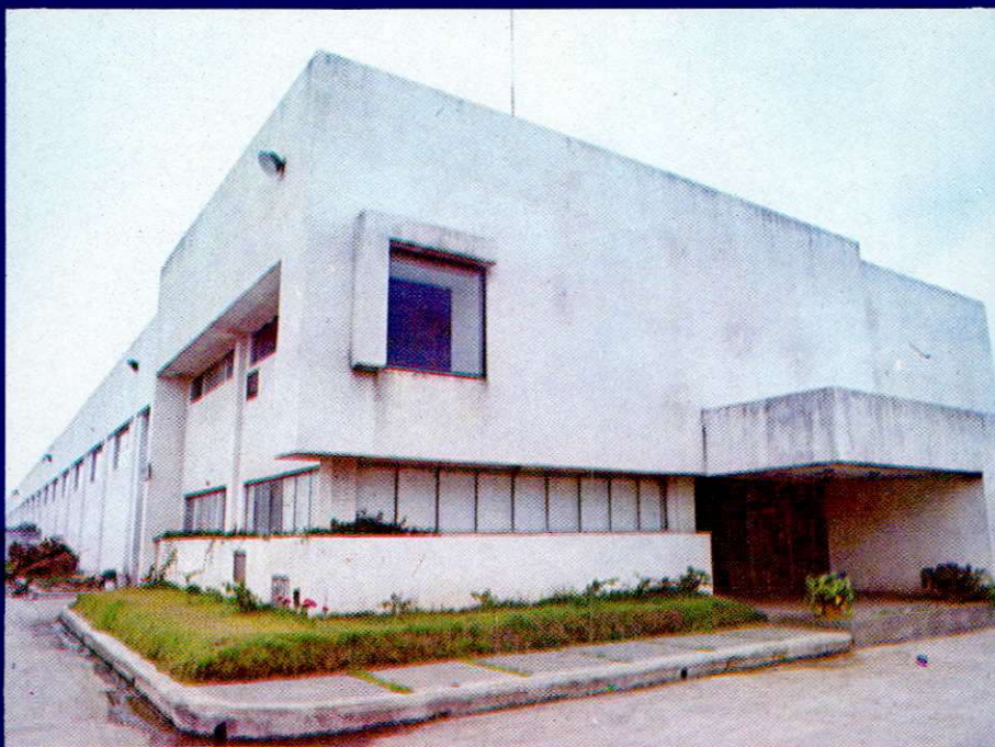
(Top) Fabrication of tubular components with elaborate designs require special engineering skills to assure adherence to dimensional tolerances. (Bottom) The Bundy Pacific Tubing (Phils.), Inc. building at Km. 40, Sta. Rosa, Laguna houses the fabrication plant.
