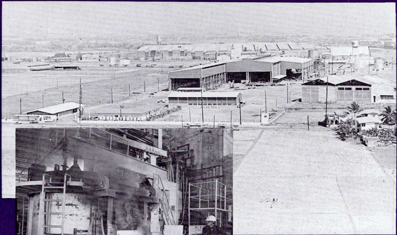
An aerial view of the Armco Marsteel steelworks in Taguig, Metro Manila. (Inset) 30 metric ton electric arc furnace in operation.
