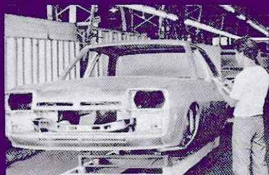
(top) Underbody assembly. (bottom left) B.I.W. obtaining "O.K." sticker from quality control. (bottom right) Unit being top coated with acrylic paint.
