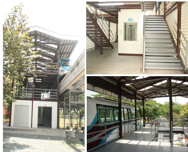
Figure 2. Completed AGT System passenger station at E. Jacinto Street (Station 1)
