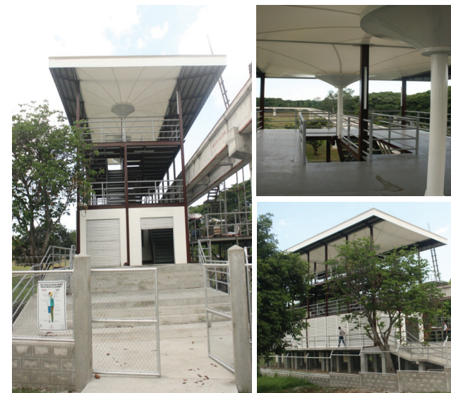
Figure 3. Completed AGT System passenger station at C.P. Garcia Avenue (Station 2)
