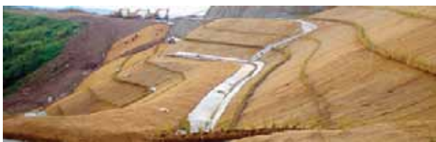
Figure 8. Biolog application on Hillside Stabilization.
