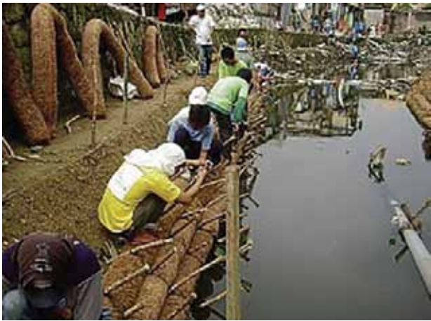
Figure 7.1 & Figure 7.2 Biolog application in river embankments.
