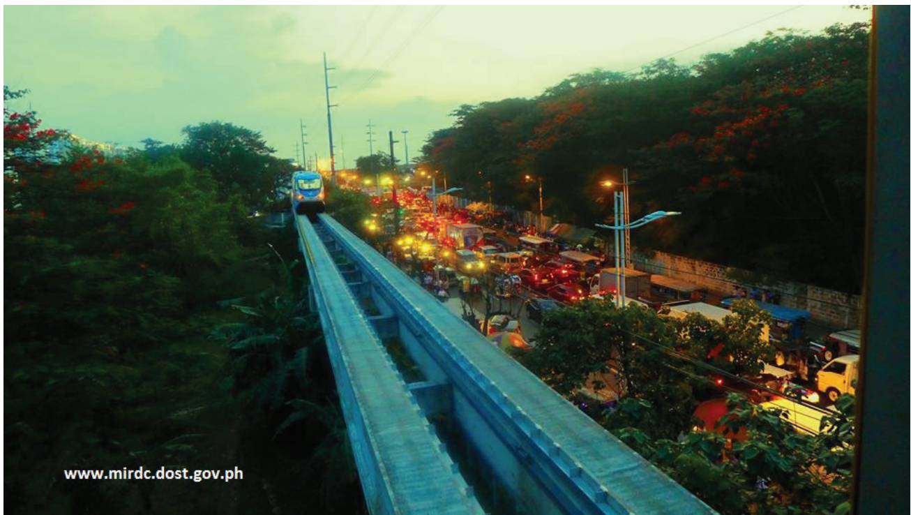
Figure 1. AGT Bicutan and the traffic situation along Gen. Santos Ave. during rush hour
