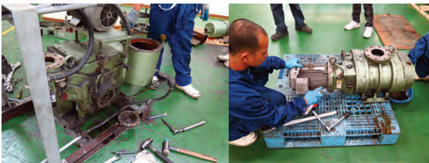
Figures 5 and 6. Assessment and overhauling of rotary pump and booster pump.
