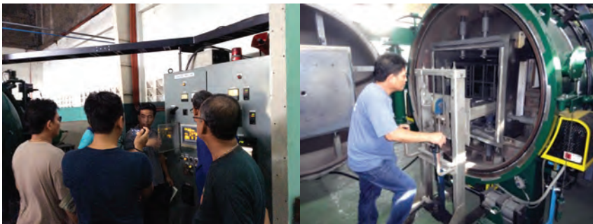
Figures 7 and 8. Orientation and training of Heat Treatment personnel on the operations of Chugai Ro vacuum heat treatment furnace.
