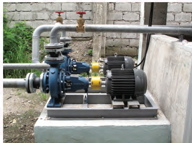
Figure 4. Installation of pumps (one as spare) for the cooling water system.
