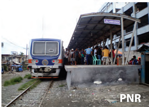
Figure 1. Current situation of railway lines in the Philippines
