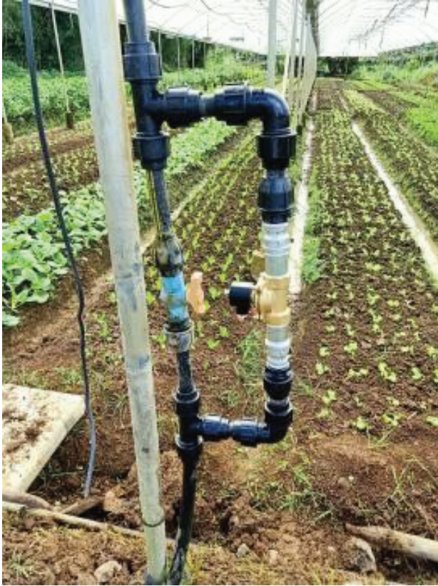
Figure 5. Solenoid Valve Bypass Setup
