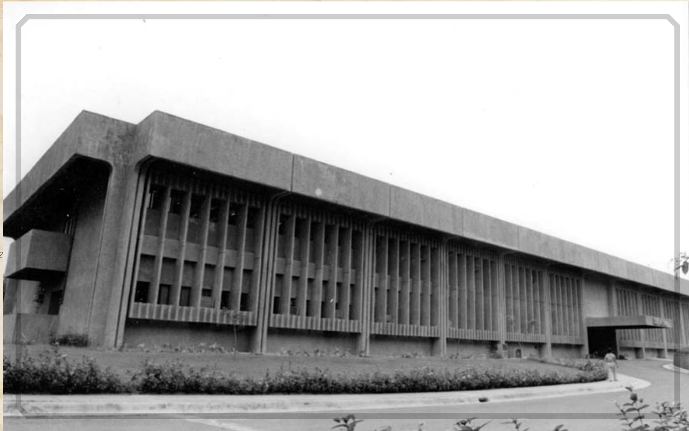
Administration and Laboratory Building
