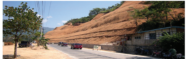
Figure 9. Biolog application on Highway slope embankment.
