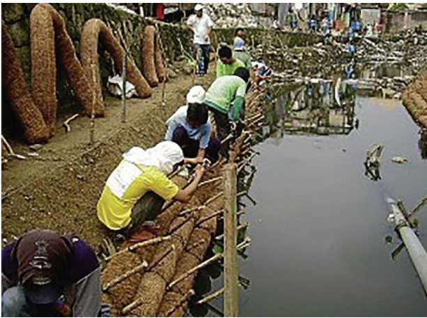
Figure 7.1 & Figure 7.2 Biolog application in river embankments.
