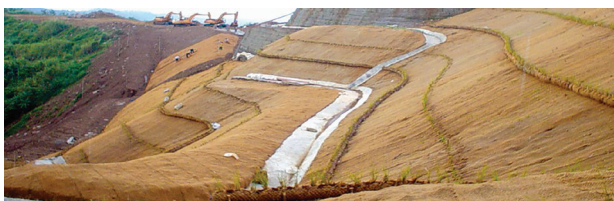
Figure 8. Biolog application on Hillside Stabilization.
